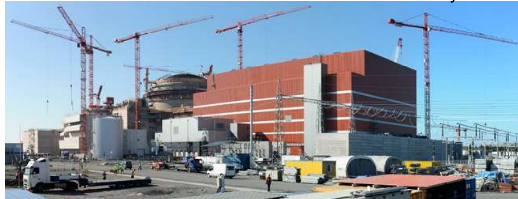
OL3 construction site in May 2010
